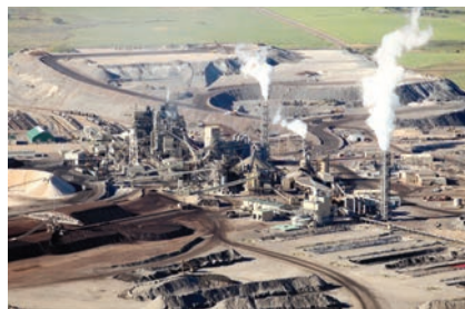
Mines and construction sites
