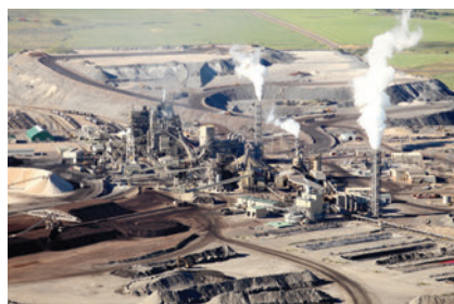
Mines and construction sites
